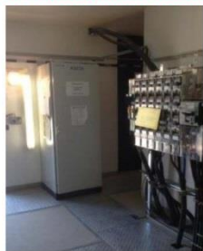
ICT-Schrank in Transformatorstation ... Transformatorstation ... Trennschlusskasten
